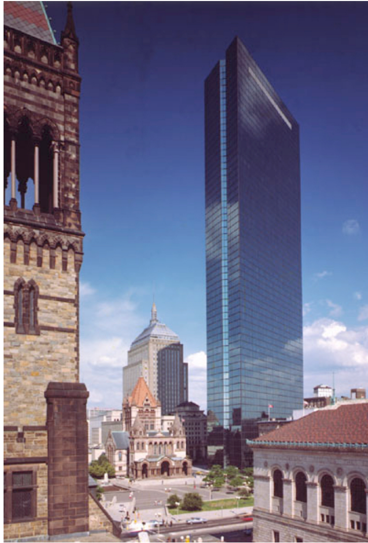
Figure 5.5.1 The John Hancock Tower
